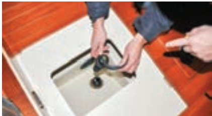
➤ This is the through-hull for the triducer. When replacing it, lubricate the O-ring with grease to prevent leaks. Make sure that the arrow is pointing in the right direction. If it's an older one with the cut out, it has to be positioned correctly or it will leak.
